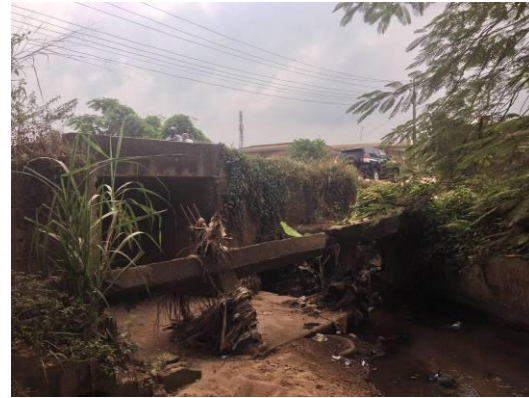
Collapsed culvert
