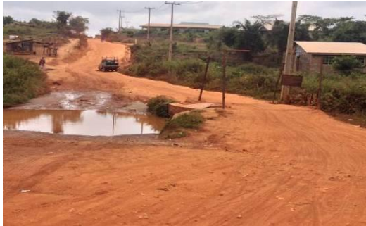
Earth road, make shift drainage forms the approach In adequate single culvert
