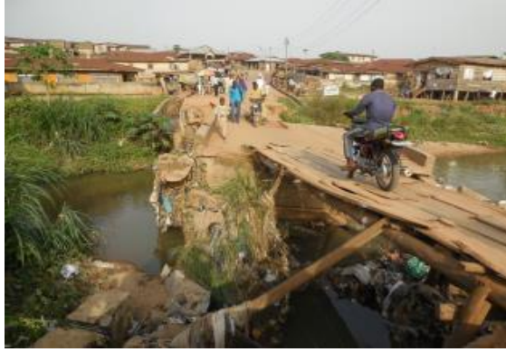
Community intervention on the collapsed bridge
