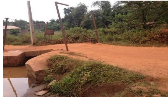
Earth road, make shift drainage forms the approach In adequate single culvert
