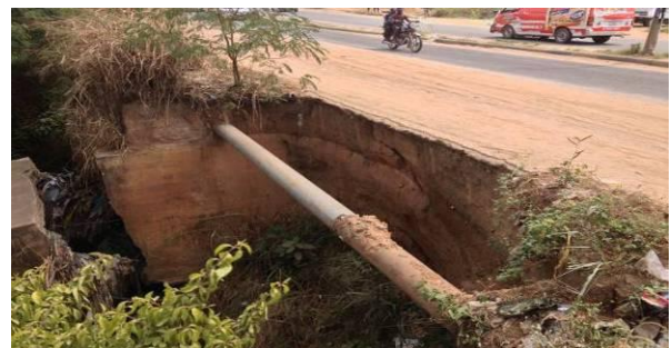
Exposed telecommunication/water utilities
