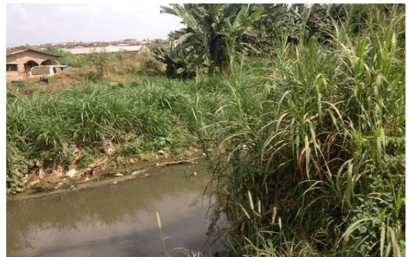
Aquatic weeds restricting flow of water
