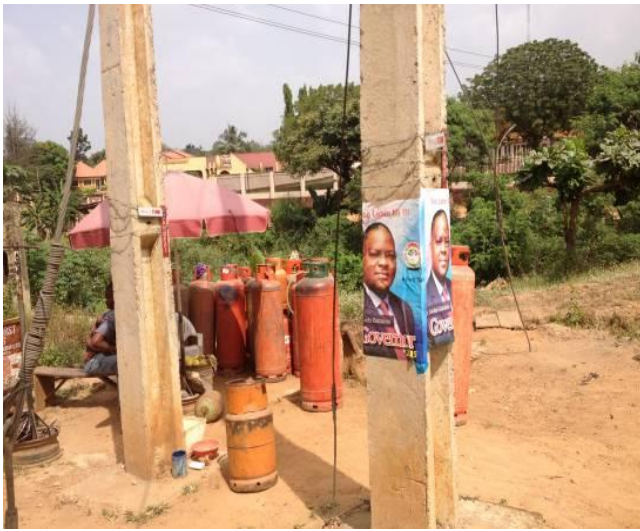
c.) Affected public utility and gas vendor
