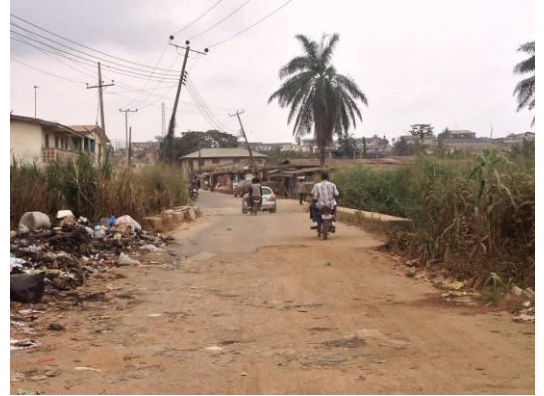
f.) Affected house close to the
