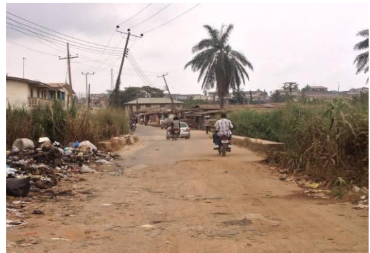
f.) Affected house close to the damaged bridge
