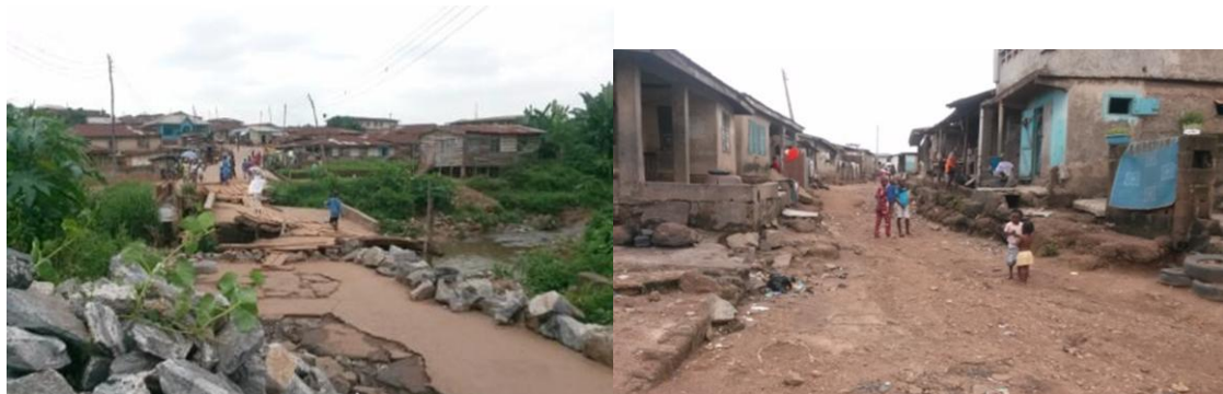
Collapsed Bridge as the major hazard in the community
