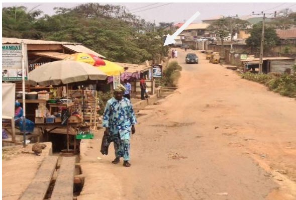
e.) Affected kiosks along the drainage way
