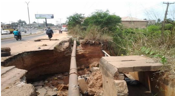
Undercutting of road; damaged drainage
