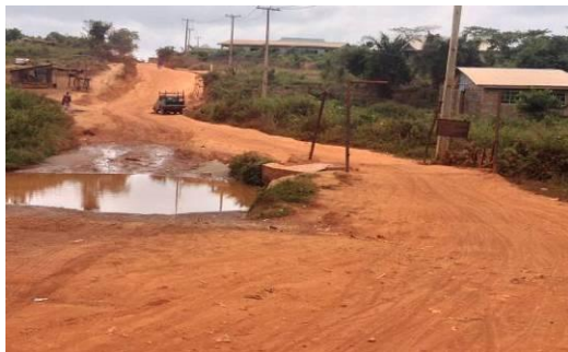
Earth road, make shift drainage forms the approach
