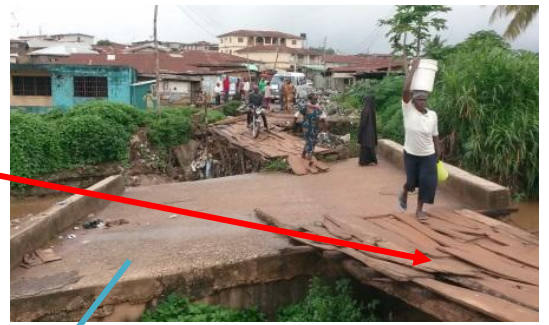
Crossing from damaged OgbereMoradeyo culvert to other side of the road using foot bridge
