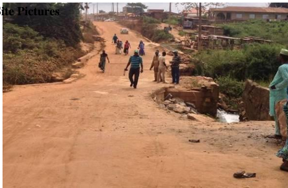
Roadway approaches; no drainages
