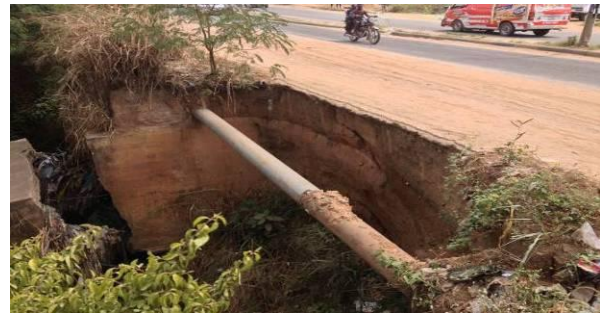
Exposed telecommunication/water utilities
