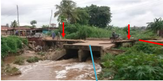
Temporary foot bridges (in red arrows) on either side of the damaged culvert, used by people to cross from culvert to both sides of the road
