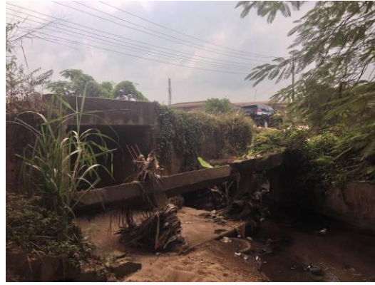
Collapsed culvert
