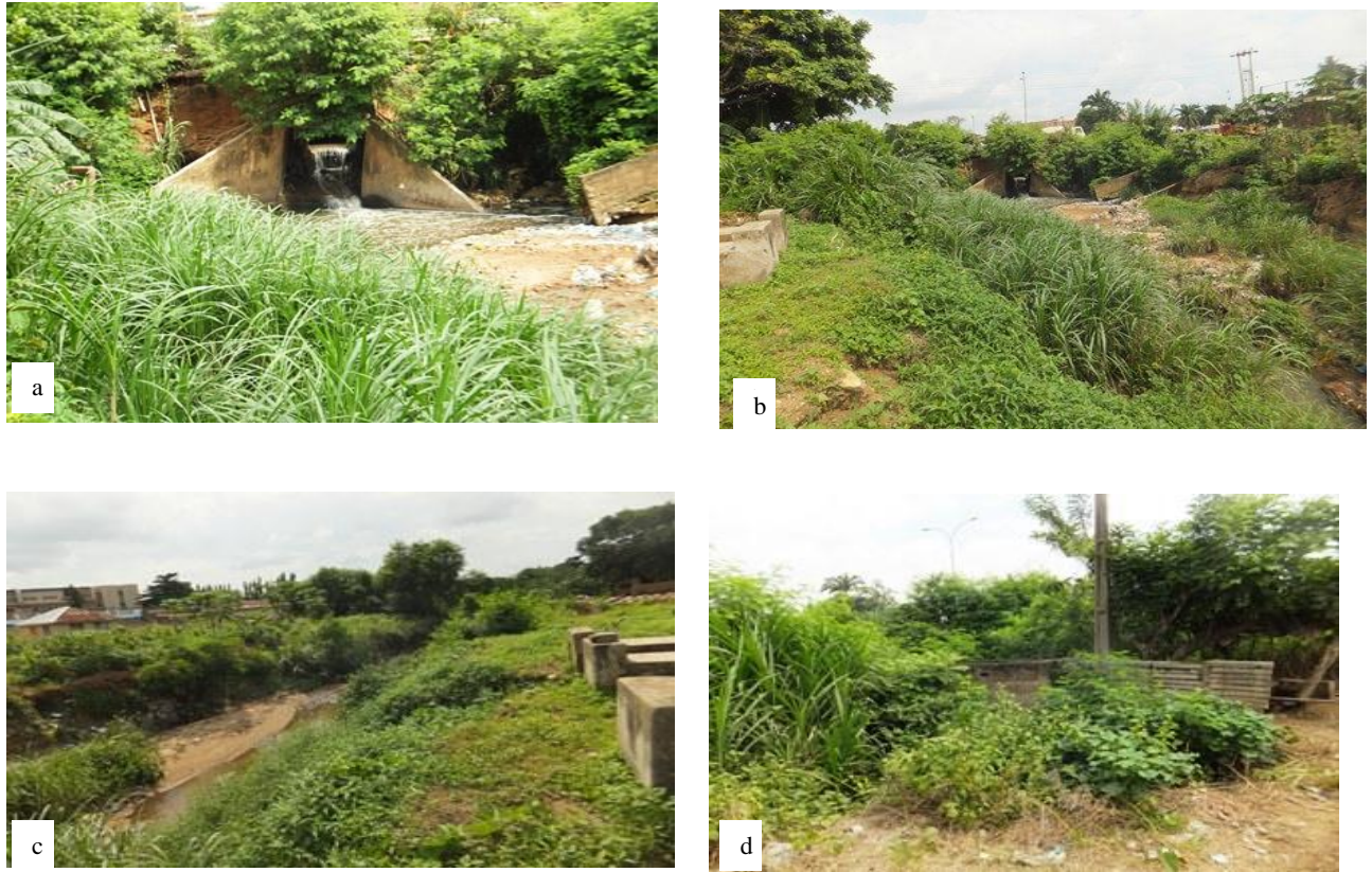
Plate 5.2 (a – d): Vegetation around Alaro Poly Culvert during Wet Season
