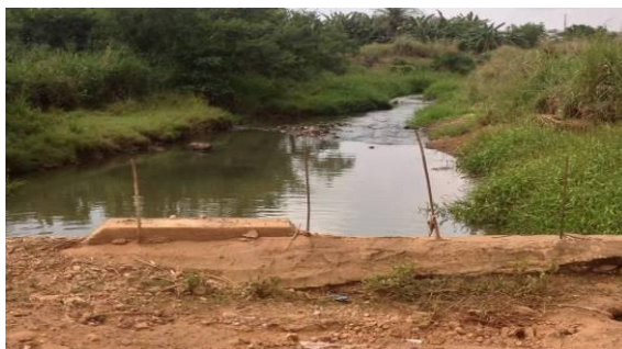
Roadway approaches; no drainages
