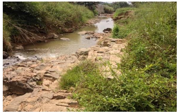
High sediment/solid waste load in stream
