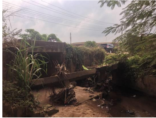
Collapsed culvert
