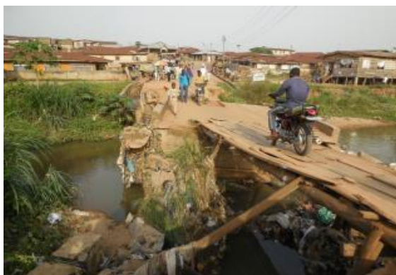
Community intervention on the collapsed bridge
