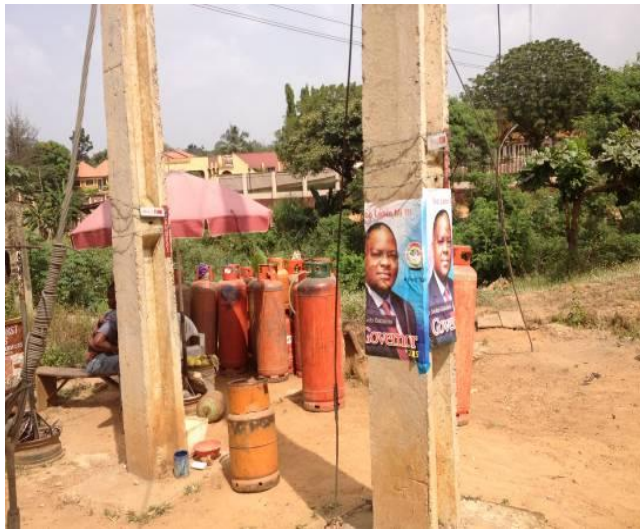
c.) Affected public utility and gas vendor
