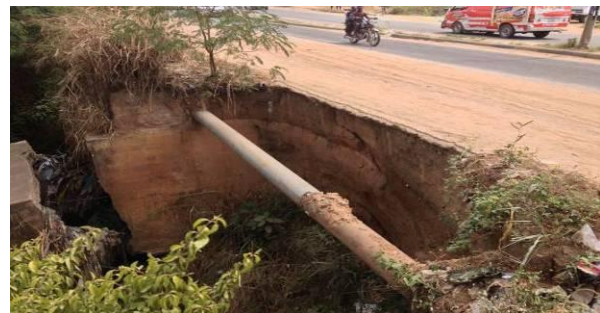
Exposed telecommunication/water utilities
