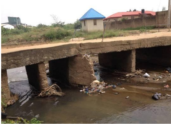
Upstream towards crossing
