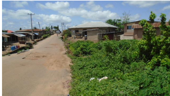
Upstream with shrubs, no drainage in place
