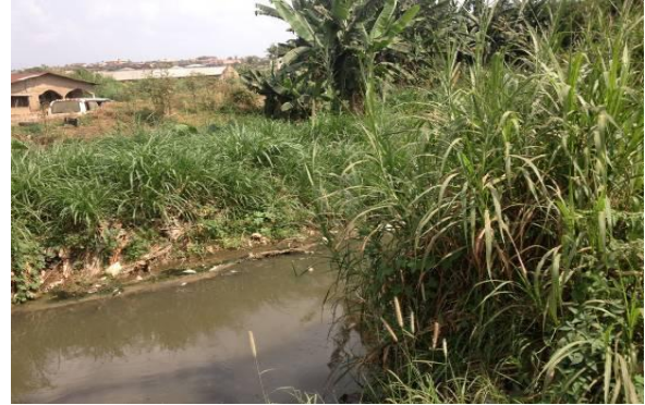
Aquatic weeds restricting flow of water
