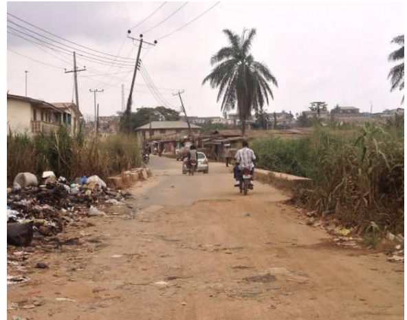
Damaged road approach; improper solid waste
