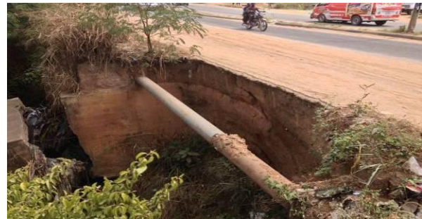
Exposed telecommunication/water utilities
