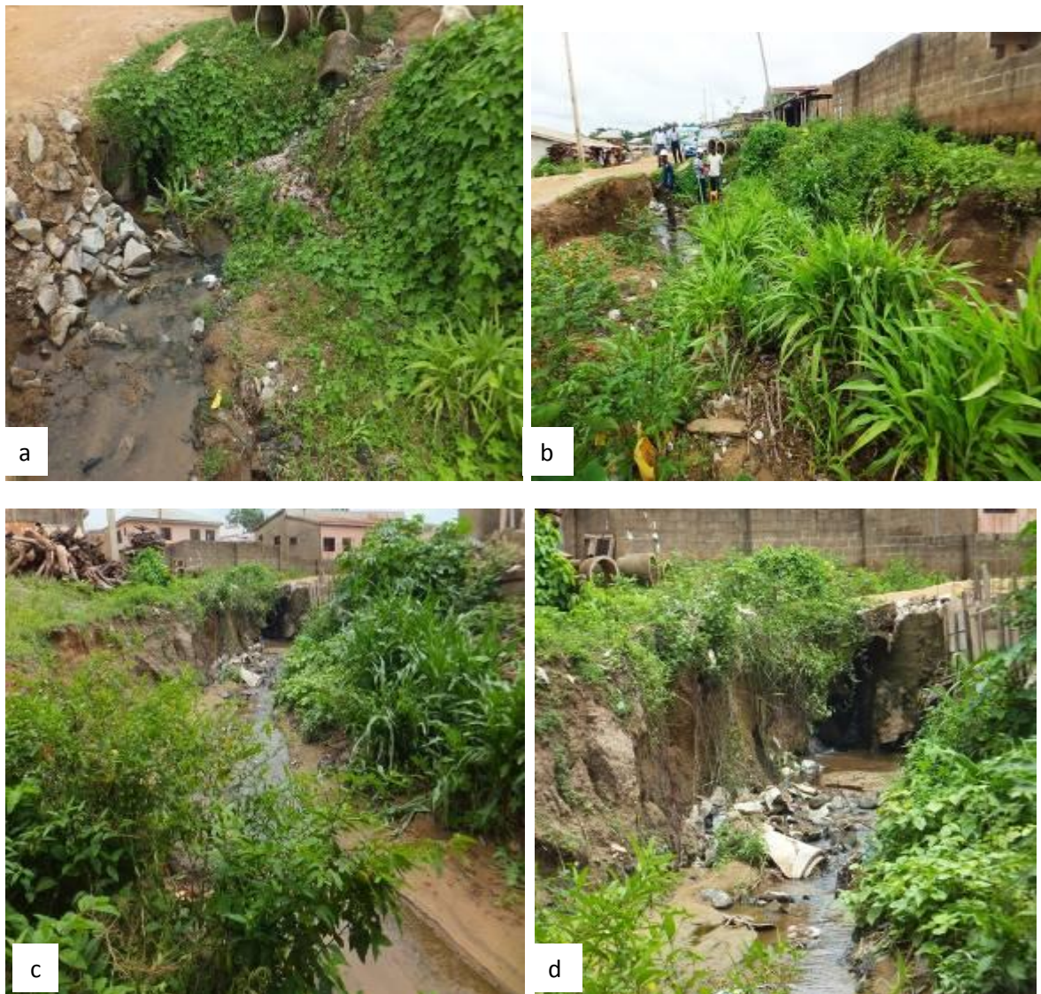
Plate 5.1(a-d): Vegetation around Olorogunwa culvert
