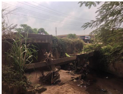
Collapsed culvert
