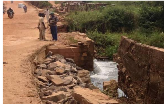
Structural damage actively eroding
