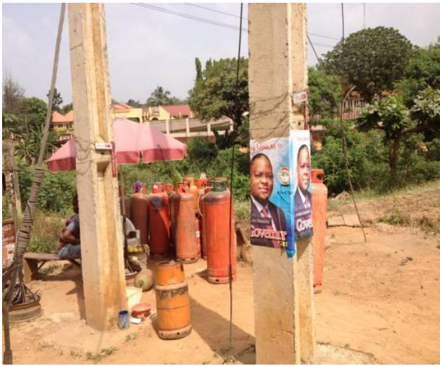
c.) Affected public utility and gas vendor
