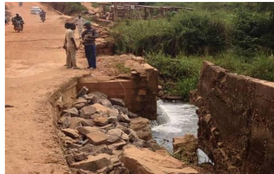
Structural damage actively eroding
