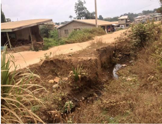
Collapsed culvert
