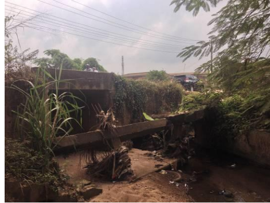
Collapsed culvert
