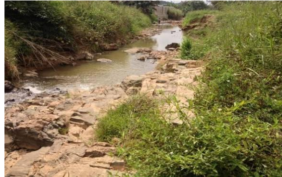
High sediment/solid waste load in stream
