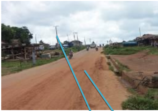
Egbeda Tuba road and PHCN (IBPD) pole
