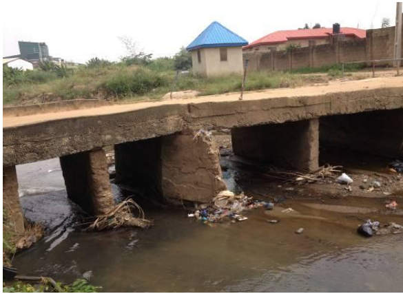
Upstream towards crossing
