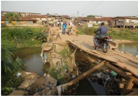
Community intervention on the collapsed bridge
