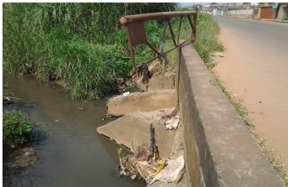
Structural damage to existing culvert
