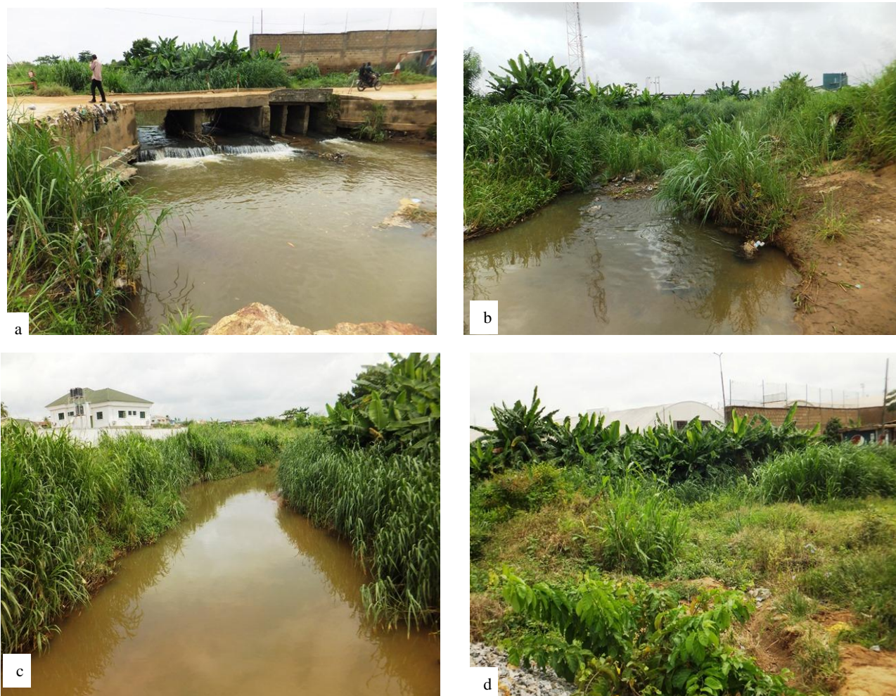
Plate 4.1(a-d): Vegetation around Alaro 7up Road Culvert.
