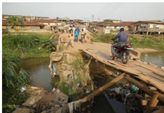
Community intervention on the collapsed bridge
