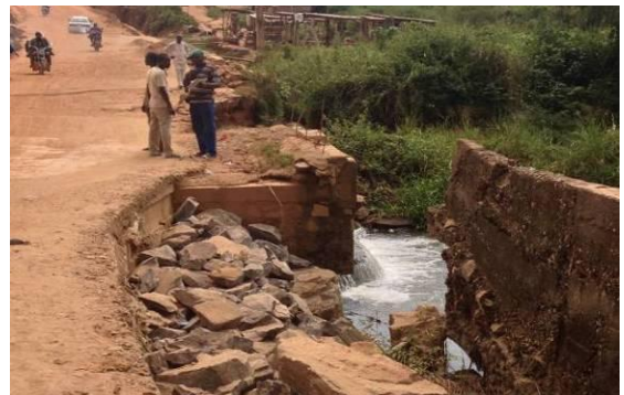
Structural damage actively eroding
