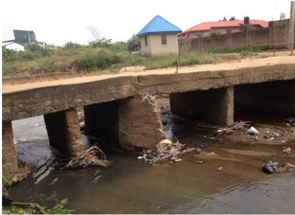
Upstream towards crossing
