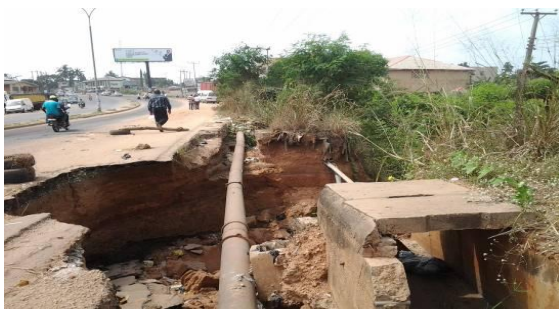
Undercutting of road; damaged drainage
