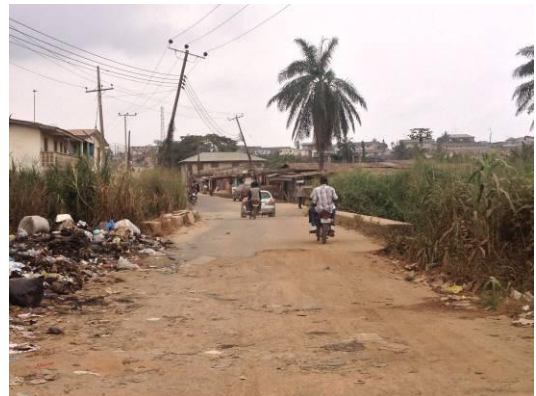
f.) Affected house close to the damaged bridge
