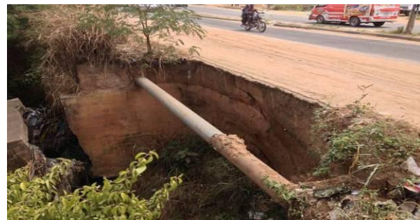
Exposed telecommunication/water utilities
