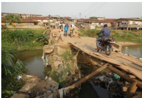
Community intervention on the collapsed bridge
