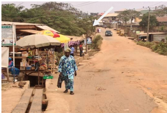
e.) Affected kiosks along the drainage way
