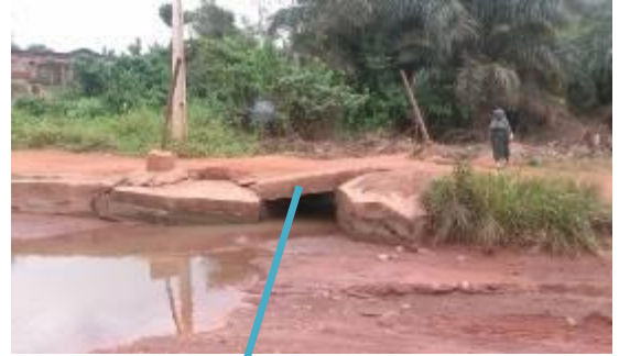
Temporary culvert made by community efforts
