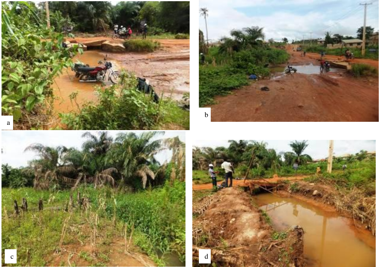
Plate 4.1(a-d): Vegetation around Elere culvert.
