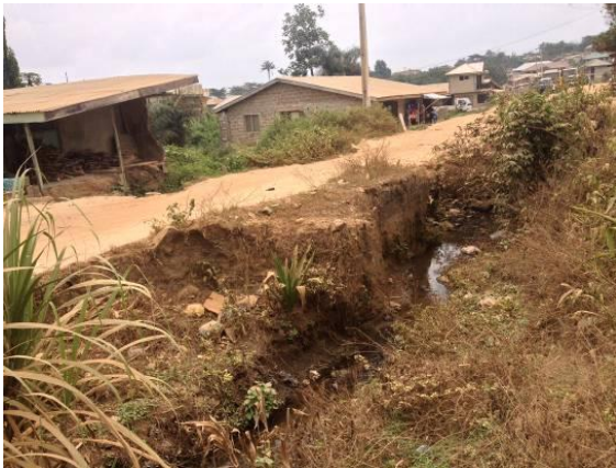
Collapsed culvert
