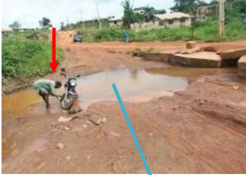
Motorbike being washed in the river, on which heavier vehicles pass (beside the temporary culvert made by the Community)
