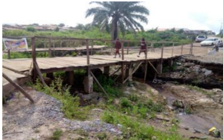
PIC 3.2 - Existing makeshift Alternative Bridge to be improved upon
