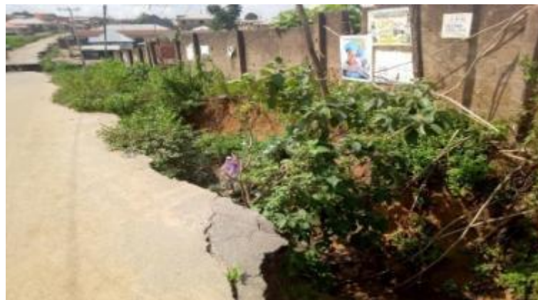
PIC 3.1 - House fence that could be affected by Drainage Reconstruction
