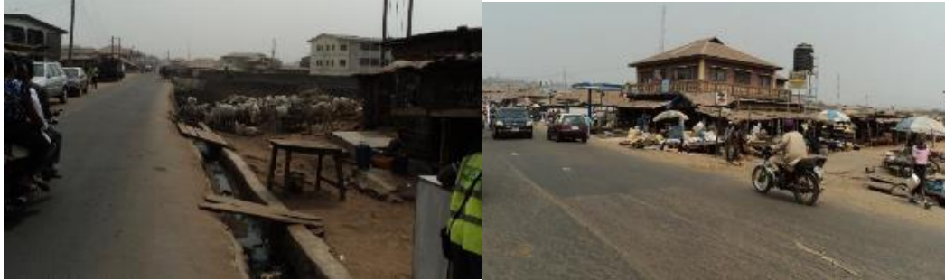
Plate 5. 7: Inter-Community Road Network (Oranyan - Labo road)
